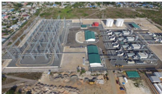
Gas Fired Power Plant
